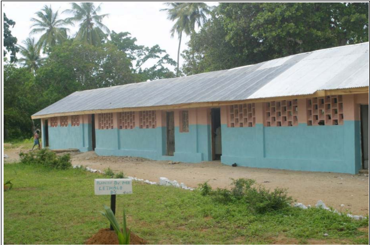
Majaoni Primary school after renovation
