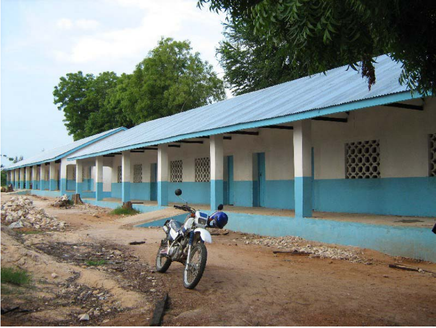
2 of the finished blocks in phase one at Chumani primary school
